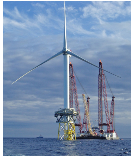
Fig. 4.30. Mounting of 5 MW wind turbine, Germany, North Sea coast
