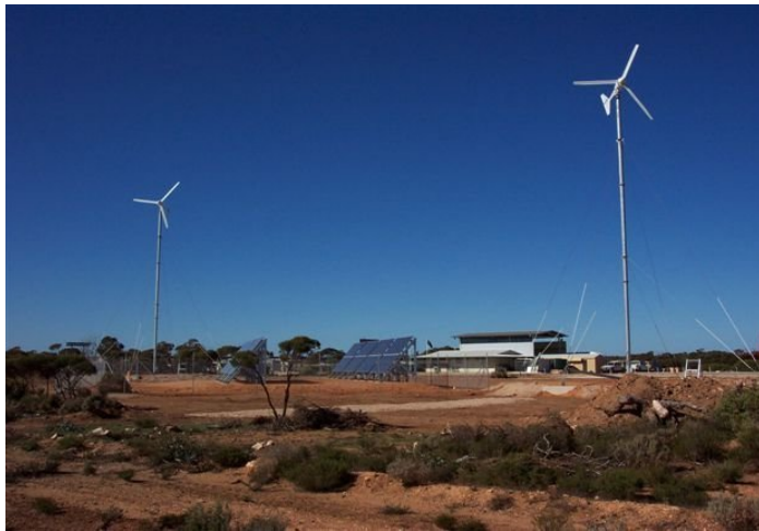
Fig. 4.39. Two WestWind 10 kW turbines installed at Euda wind farm (Australia) [40]
