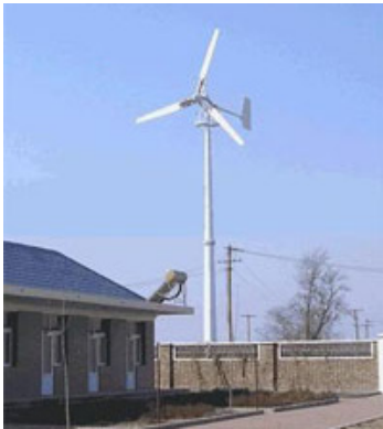
Fig. 4.41. 10 kW Tairui wind turbine.
